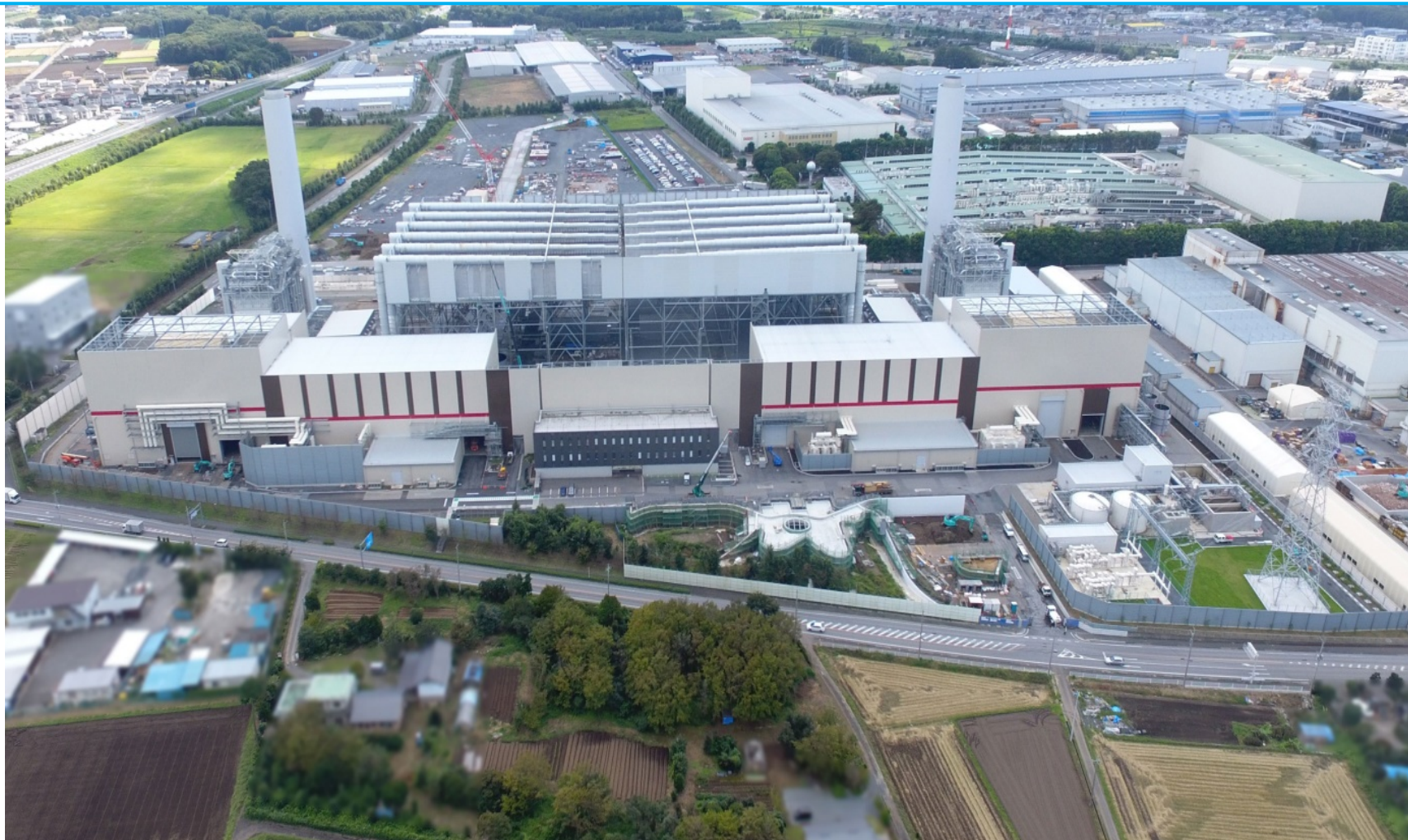
The Moka Power Plant (taken in September 2019)
