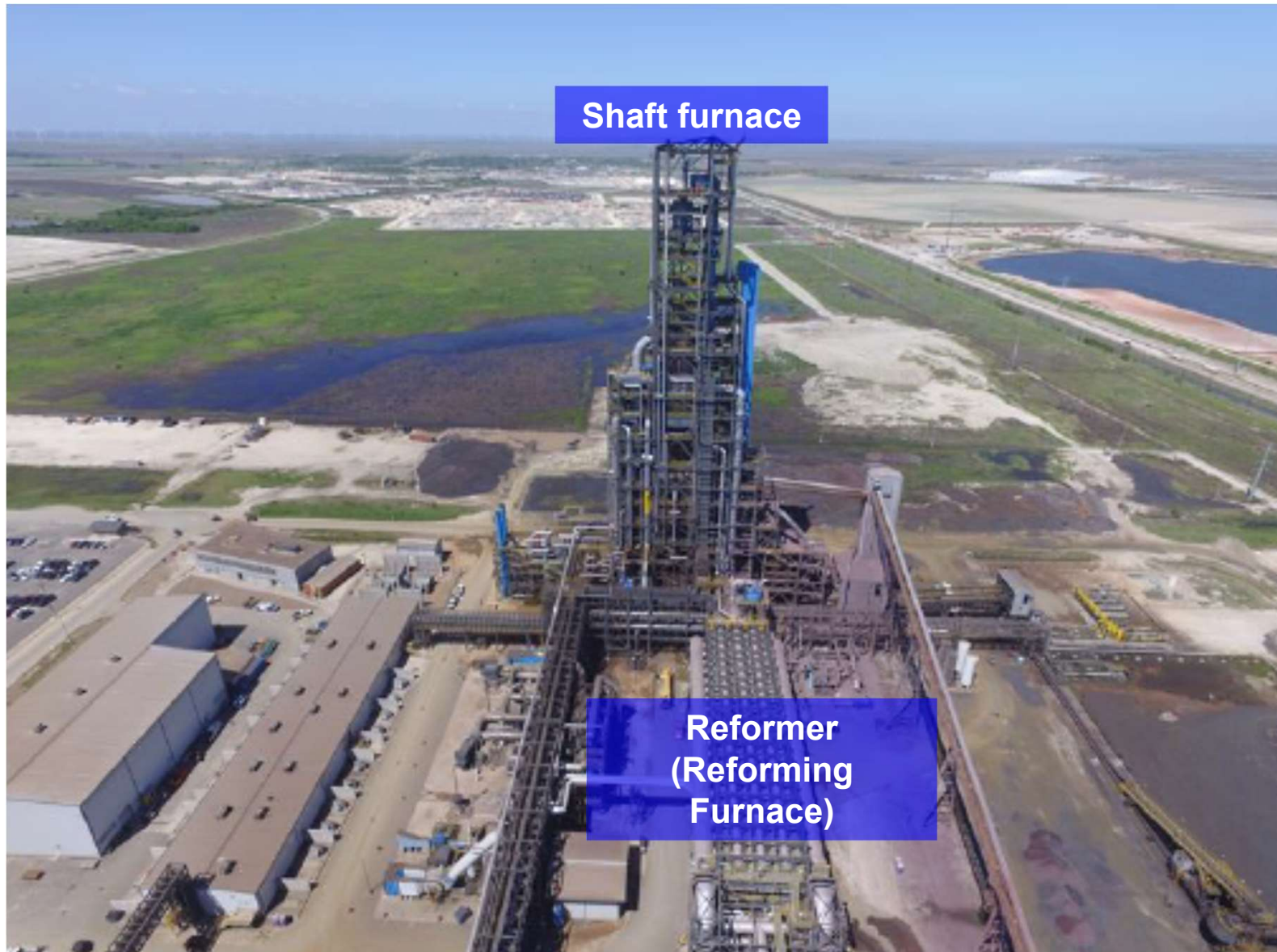
“Go West” Plant, voestalpine (U.S.A.) (2 Mt/year)
