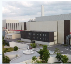
Moka Power Plant
