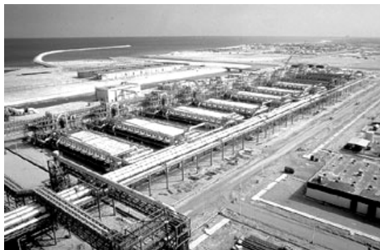
Photo 1.4 A seawater desalination plant (Photo courtesy of Hitachizosen Co., Ltd., Japan)
