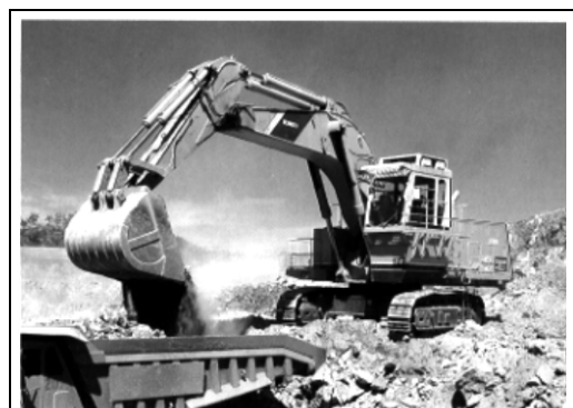
Photo 2.1 — A hydraulic excavator in operation on a rocky-soil ground
