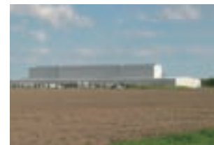
Continuous annealing facility at PRO-TEC now in operation
