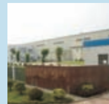
Kobe Wire Products (Foshan) Co., Ltd.
