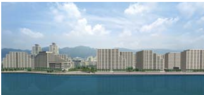
Maya Seaside Place, a condominium development in eastern Kobe
