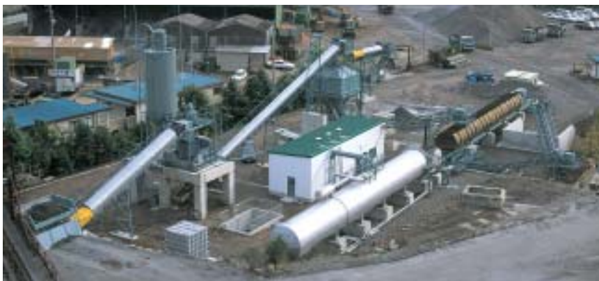
The Ecosand Recymer is the world's first commercial waste sludge stabilization and treatment system. Stabilizing dry rock dust, construction sludge or dredged sludge, the plant produces artificial sand, which can be used in concrete, or formed products, such as interlocking blocks. By using stabilized waste sludge, the system contributes to improving the environment.
