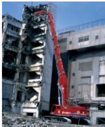
Ultra long attachments can demolish over 50 m tall buildings, the highest in its class. This SK 1600D reduces noise and vibration at the work site.
