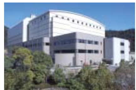
This solid waste treatment plant in Kakogawa in western Japan helps lessen the burden on the environment. We also supply wastewater treatment plants and are broadening our environmental menu.
