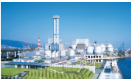
With the start-up of the second of two plants, the Shinko Kobe Power Station is now in full operation.
