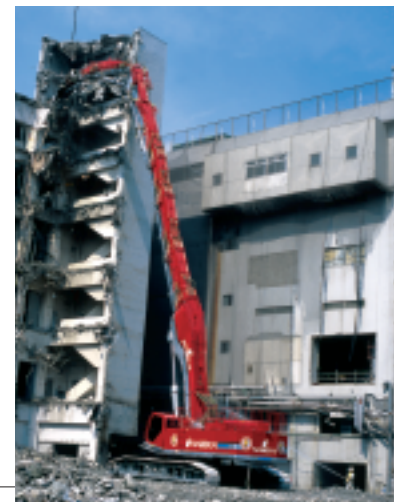
The SK 1600D can demolish buildings over 50 meters tall. The ultra long boom gives this machine one of the highest reaches in its class.
