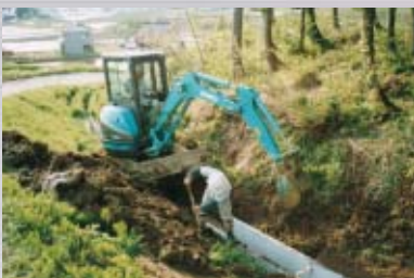
■ A Kobelco mini excavator is used to help rebuild water supplies after the Niigata Chuetsu earthquake.
