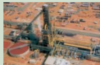
Direct reduced iron plant in Venezuela
