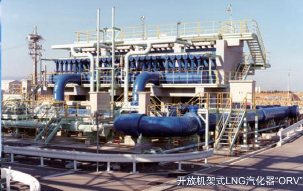
开放机架式LNG汽化器“ORV”
