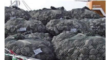
Submerged breakwater construction material (Filling material: steel slag hydrated matrix)
