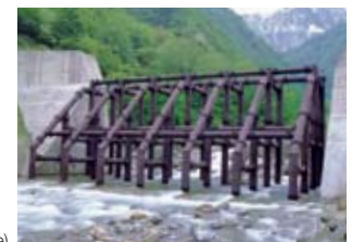
Sediment control dam on Ikazawa River (Niigata Prefecture)
