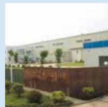
Kobe Wire Products (Foshan) Co., Ltd.
