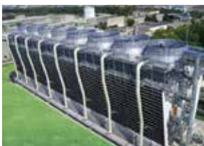
Plume abatement cooling towers
