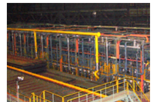
New heat treatment furnace
