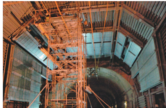
Fig.12 Installation of microperforated panels
