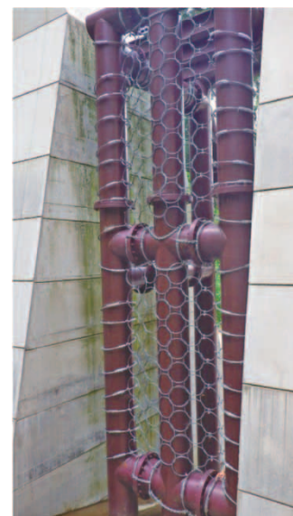
Fig. 9 A completed GRID NET
