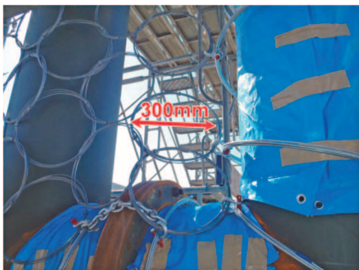
Fig. 7 Attachment of the mesh of rings
