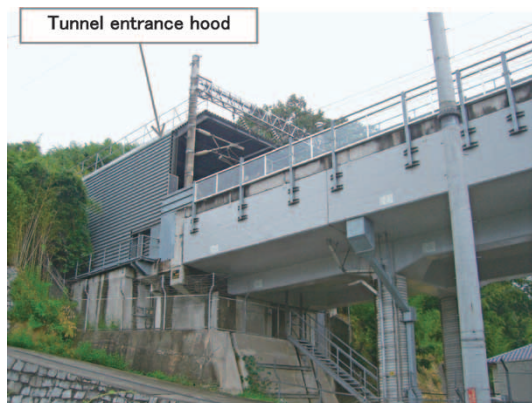
Fig. 3 Tunnel entrance hood for Shinkansen
