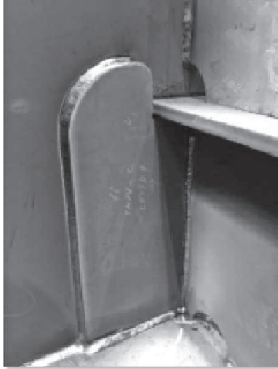
Fig.10 Robotic welding result B
