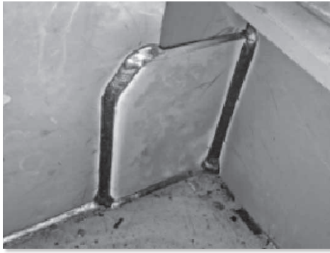
Fig. 9 Robotic welding result A
