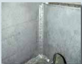
Vertical position weld appearance ①
