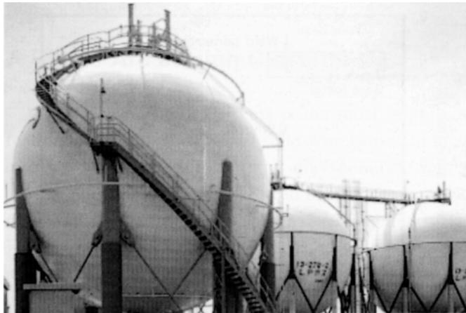
**Fig. 1 — Some types of LPG storage tanks use ASTM A537 Cl-2 steel having a minimum tensile strength of 550N/mm<sup>2</sup>, and LB-62L is one of the most suitable covered electrodes for this steel.**
