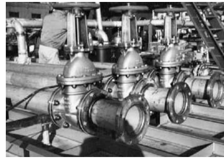
Figure 5: Stainless steel pipelines mounted on the deck of a chemical tanker
