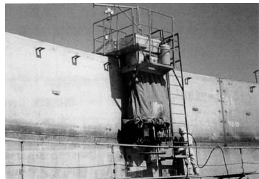
Figure 3: Application of horizontal submerged arc welding (Photo source: KHK, Safety & Tomorrow, Mar. 2000)
