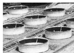
P3-7 Welding of crude oil storage tanks
