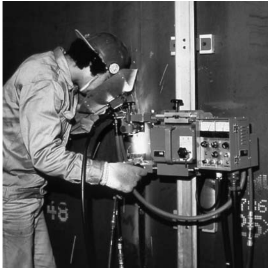
Figure 6: SEGARC process: a portable EGW process for vertical welding
