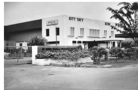
Figure 20: A production base established by Kobe Steel and Sitt Tatt in Malaysia.
