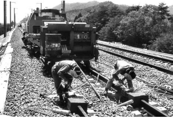
Figure 3: The long rails of the Shinkansen Super-Express Line were successfully welded by the enclosed arc welding process developed by Kobe Steel.
