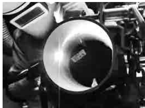
Figure 1: Site welding by TG-X filler rod
