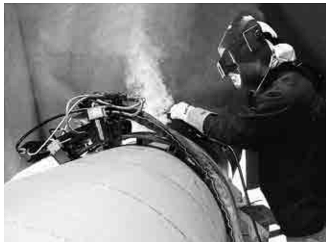
Figure 6: Welding of clad pipe by DW-N625P and Magnatech machine. Photograph supplied, courtesy of Magnatech International B.V.
