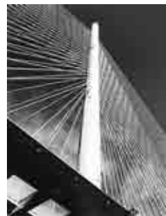
Photo 3: Stonecutters Bridge main tower, rising over 175 m above sea level (Hong Kong)
