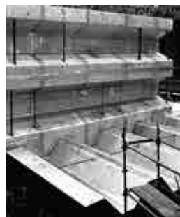
Photo 2: Chemical Tanker Bulkhead
