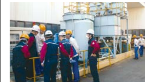
On-site environmental audit (South Korea)
