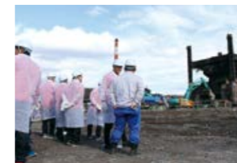
Visit to the site where the No. 3 Blast Furnace at Kobe Works, once called a symbol of reconstruction, was being dismantled
