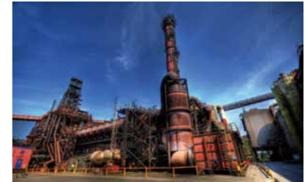
ArcelorMittal's existing direct reduction plant at its steelworks in Hamburg, Germany
