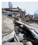
After the earthquake
