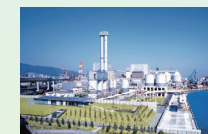
Kobe Power Plant No. 1 and No. 2 units
