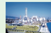
Kobe Power Plant No. 1 and No. 2 units
