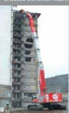
The SK3500D demolition machine has a maximum reach of over 65 meters. The SK3500D is recognized in the Guinness Book of Records as the demolition machine with the longest high reach in the world.
