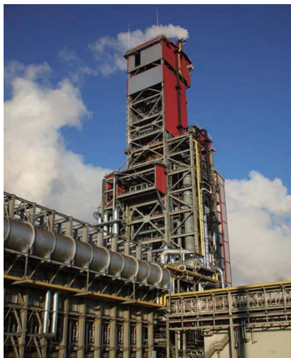
A direct reduction plant using the MIDREX® Process for the Lebedinsky Mining and Processing Integrated Works in Russia
