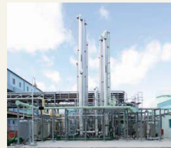
Biogas Upgrading System
