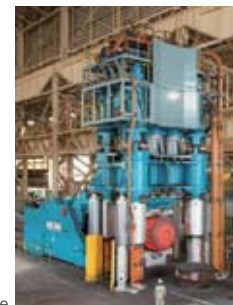
Completed new press line
