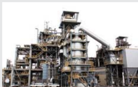
Nittetsu Shinko Metal Refine's steel mill dust recycling plant
