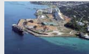
Shipping port: Port of Albany
