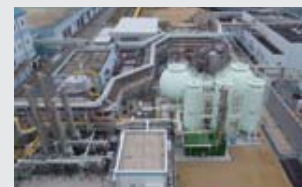
Demonstration facility for Kobe Green Sweets Project (Photo courtesy of Kobe City Construction Bureau)
