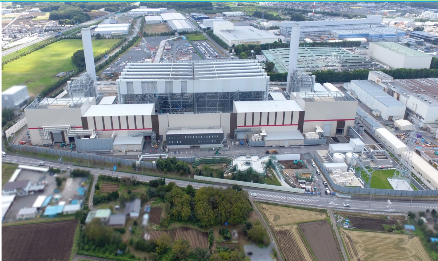
The Moka Power Plant (taken on September 2019)
