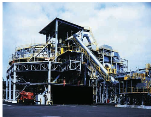
Fig. 3 No. 1 FASTMET plant in Nippon Steel Hirohata Works
