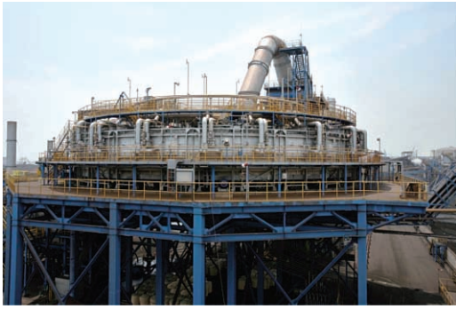
Fig.13 FASTMET plant in JFE Steel West Japan Works (Fukuyama)
