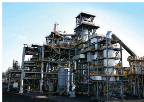
Fig. 5 No. 3 FASTMET plant in Nippon Steel Hirohata Works
