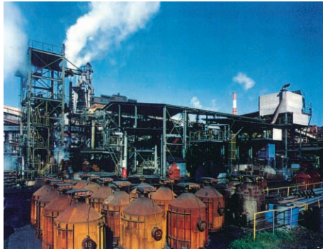
Fig. 9 Kakogawa HBI pilot plant
