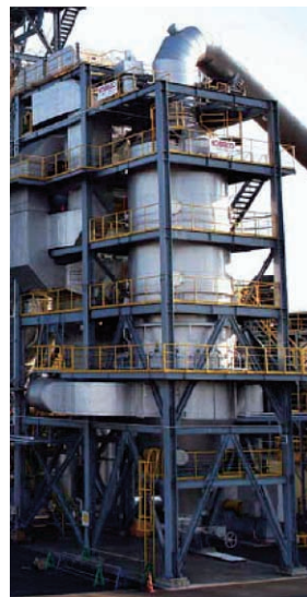
Fig.12 Exhaust gas cooler of No. 3 FASTMET plant in Nippon Steel Hirohata Works
