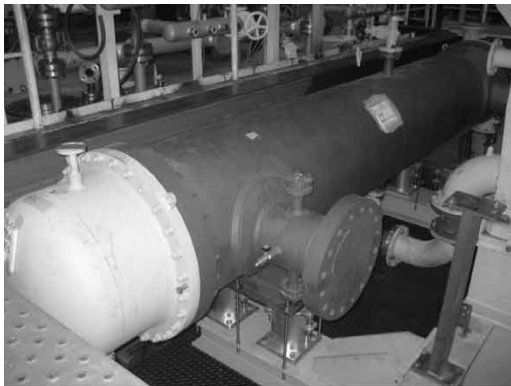
(a) Shell & Tube \Phi 650 \times 4,200 TL-TL (5,500kg)
