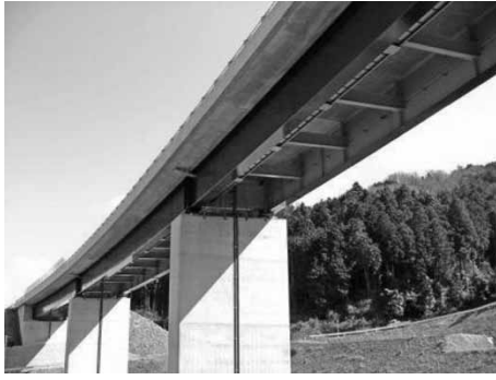
Fig. 2 Takeuchi-bashi Bridge of Minami Hanna Road
