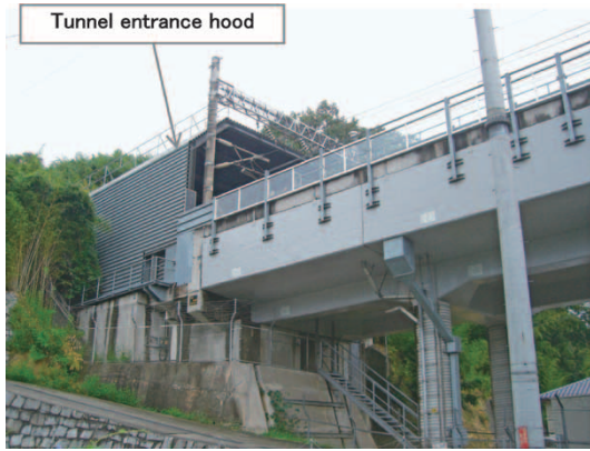
Fig. 3 Tunnel entrance hood for Shinkansen
