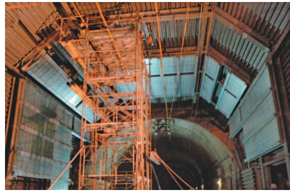
Fig.12 Installation of microperforated panels
