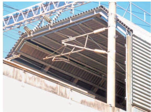
Fig.13 Microperforated panels covering inner walls of tunnel entrance hood
