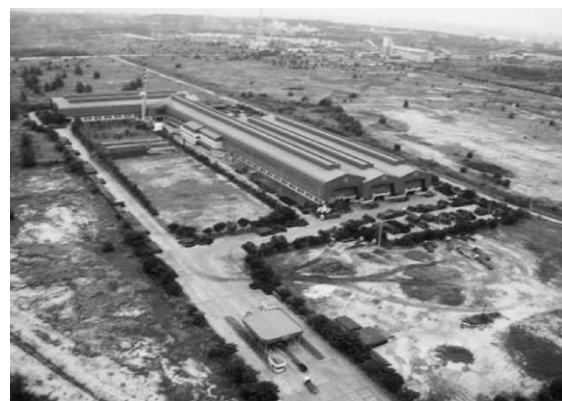
Fig. 5 Kobelco Millcon Steel
