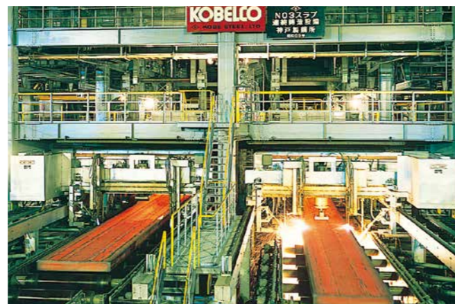
Continuous casting facility (outlet side)
