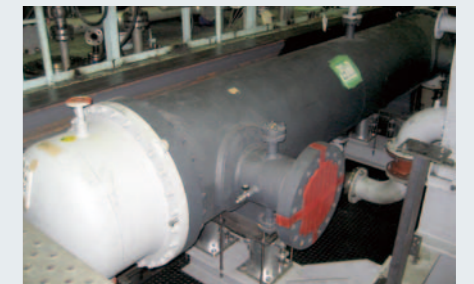
Multitubular heat exchanger Φ650×4200TL-TL (5500kg)
