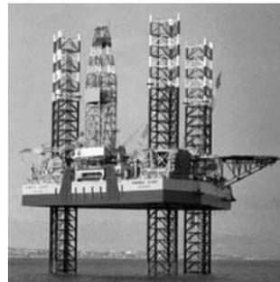
Figure 5: A jack-up rig is a typical construction that requires high performance filler metals with high impact toughness and low crack susceptibility. (Photo courtesy of Kansai Design Co., Ltd., Japan)
