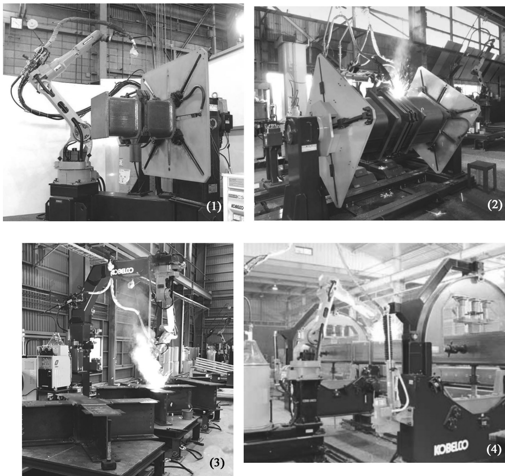
Fig.13 Steel frame welding systems using "ARCMAN™" robots for column assembly
