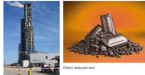
voestalpine's direct reduction plant in the U.S. in operation since mid-2017
