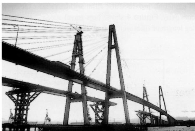
Fig. 1 — Consumption of 590N/mm<sup>2</sup>-class high strength steel is less than that of mild steel and 490N/mm<sup>2</sup>-class high strength steel, but it is an indispensable grade of steel in bridge construction, hence MG-60 is, too.
