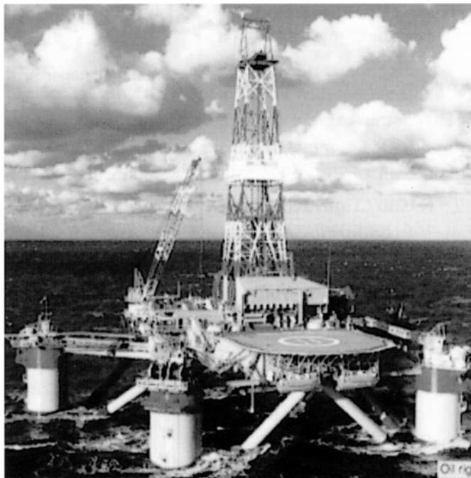
Fig. 1 — Offshore structures require strict notch toughness in order to endure operations in harsh weather and roaring waves.
