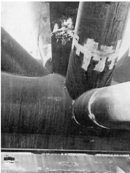
Photo 1 Node joints of a jacket
