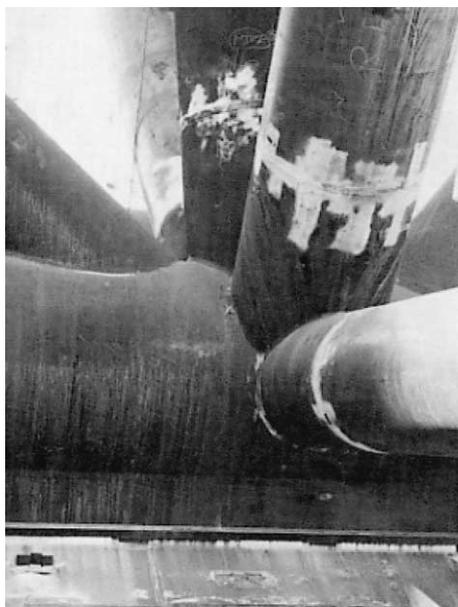
Photo 1 Node joints of a jacket
