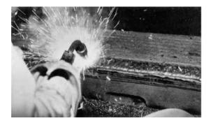
Figure 10: A typical application for **DWH-16** flux-cored wire of the high-Mn austenite type: a hot shear bite of med.C-1%Cr-Mo steel.
