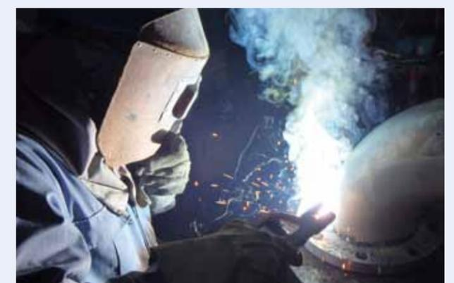
Figure 10: Welding a water pipe with **Z-1Z**
